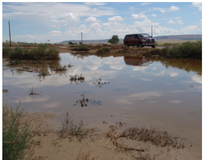
An intense storm on July 28, 2010, resulted in damage across Hopi and Navajo lands. A flash flood ruptured this sewer line near the Hopi village of Polacca. Photo: Richard Alun Davis, KUYI Hopi Radio
